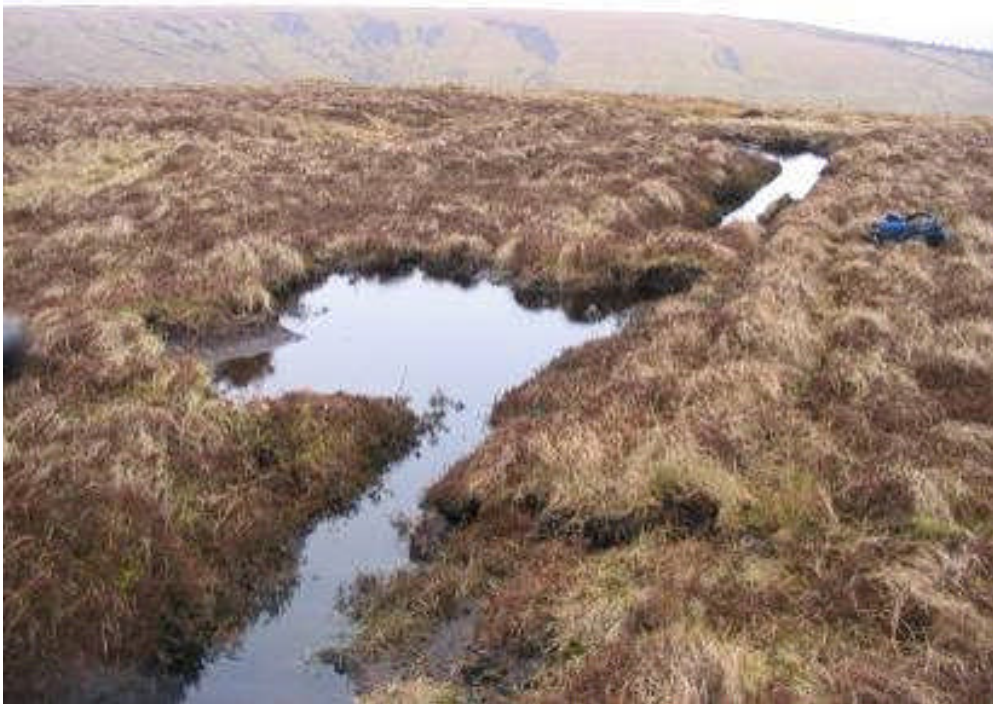
A successfully blocked peat grip in the Pennines
